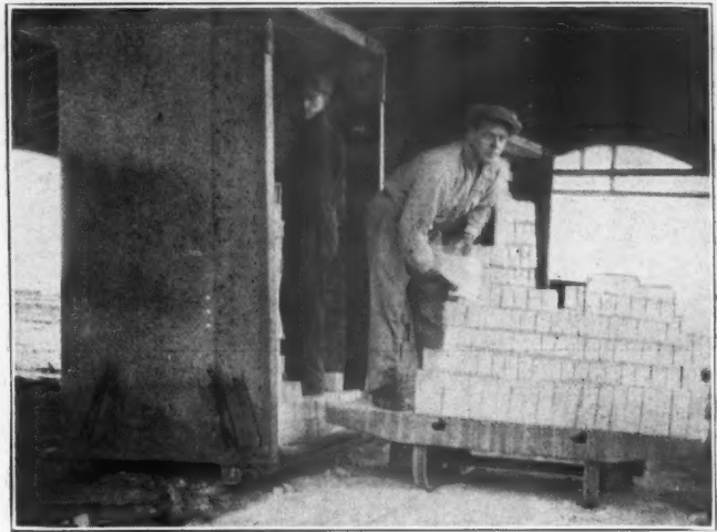
Unloading Brick Trucks Directly Into Demountable Truck Bodies
